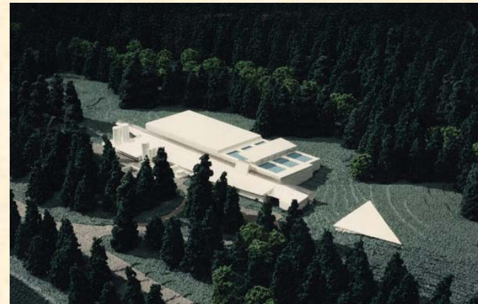
Tolt Water Plant, Seattle, WA
