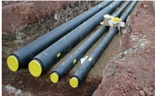
New heating and cooling system
