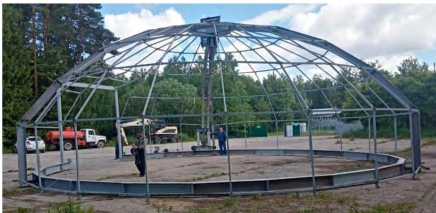
Multifunctional mobile structure with overhead polar crane
