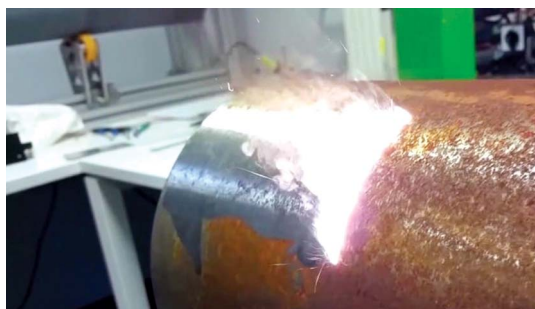
The process of laser cleaning of the pipe surface from rust
